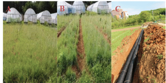
Fig. 1. The different drainage system before planting in grape orchard. A: control, B: conventional drainage, C: under drainage.
